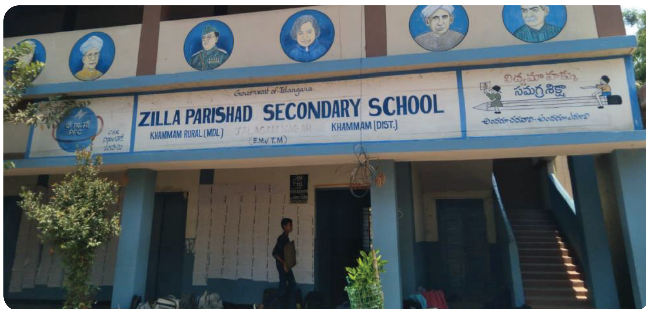
PFC constructed additional classrooms at ZPHS High School, Jagalamnagar
