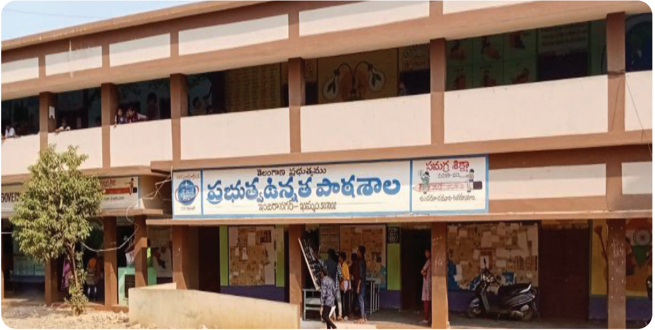
PFC constructed additional classrooms at GHS-Indiranagar Colony
