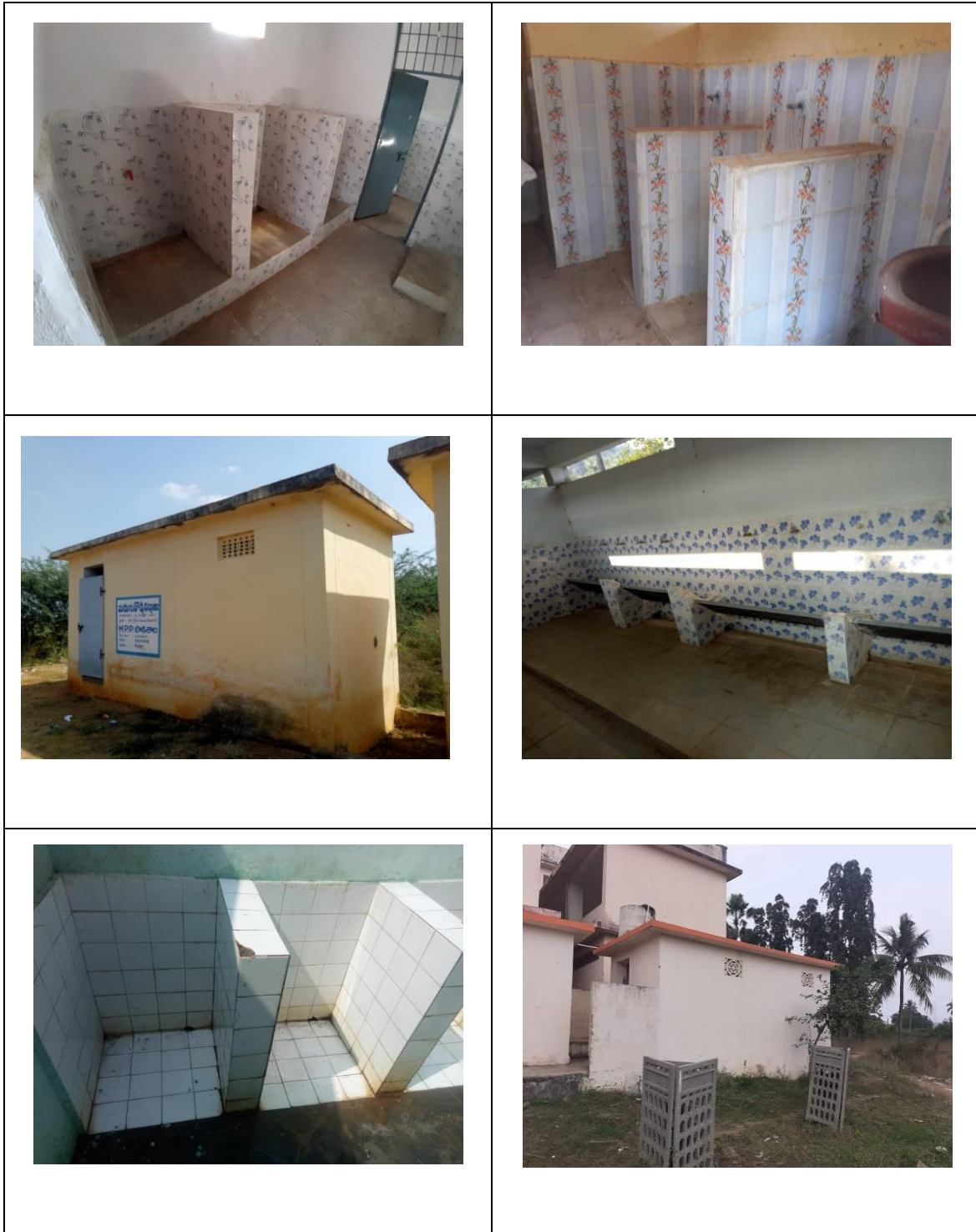
Photo 005: Sample photo of Toilet constructed in conventional method
