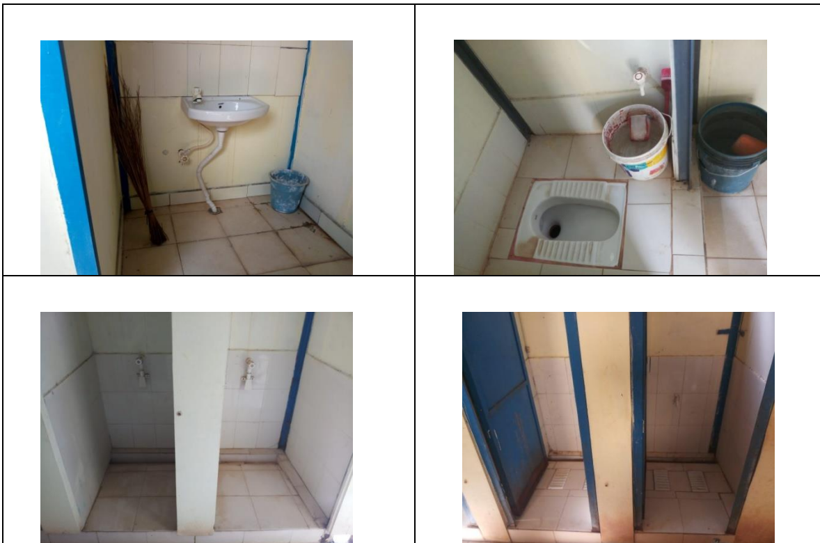
Photo 008: Sample photo showing maintenance of Toilets
