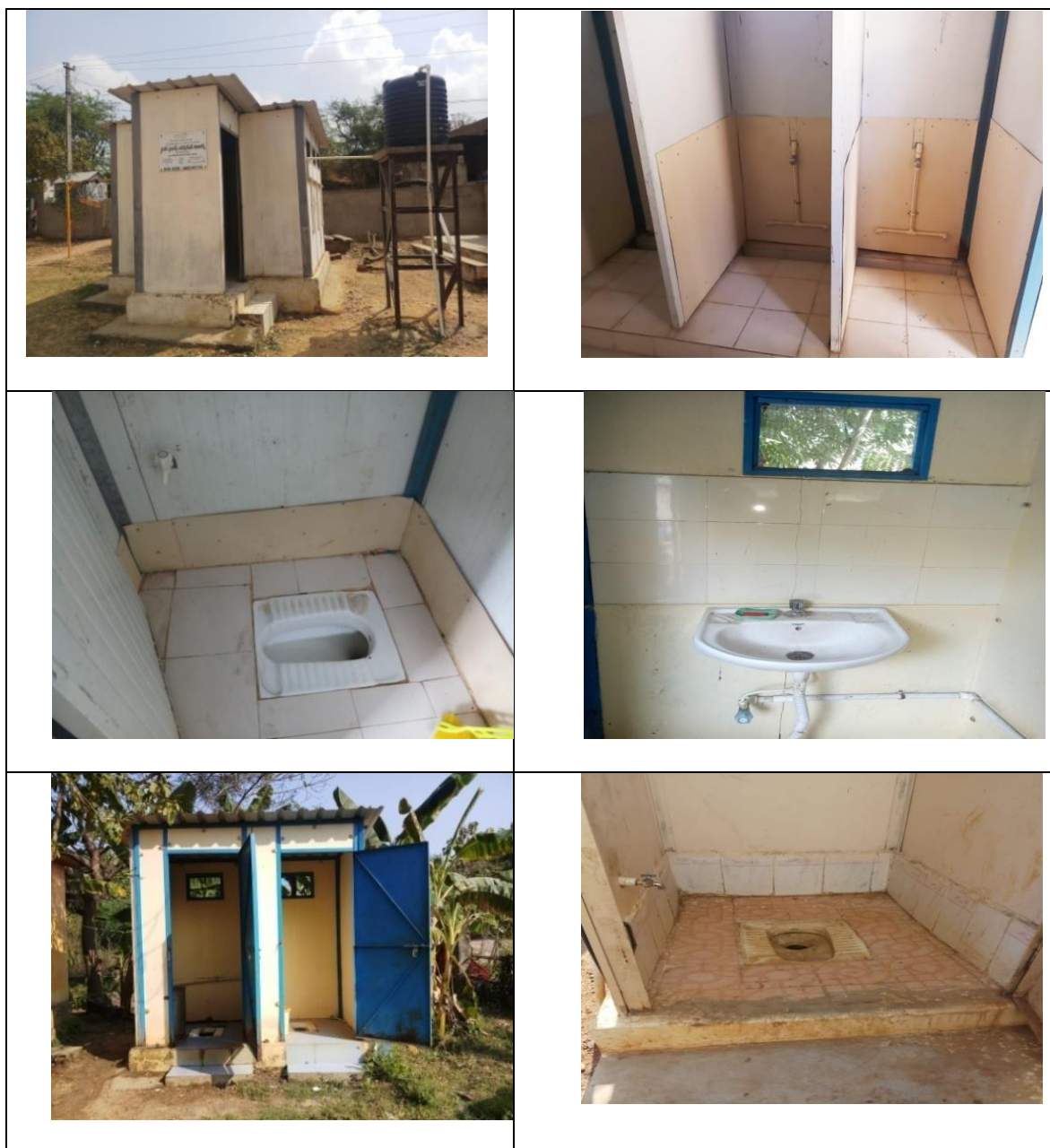
Photo 006: Sample photo of Prefabricated Toilet
